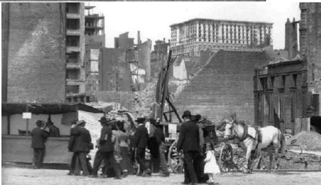
Market Street near Taylor
