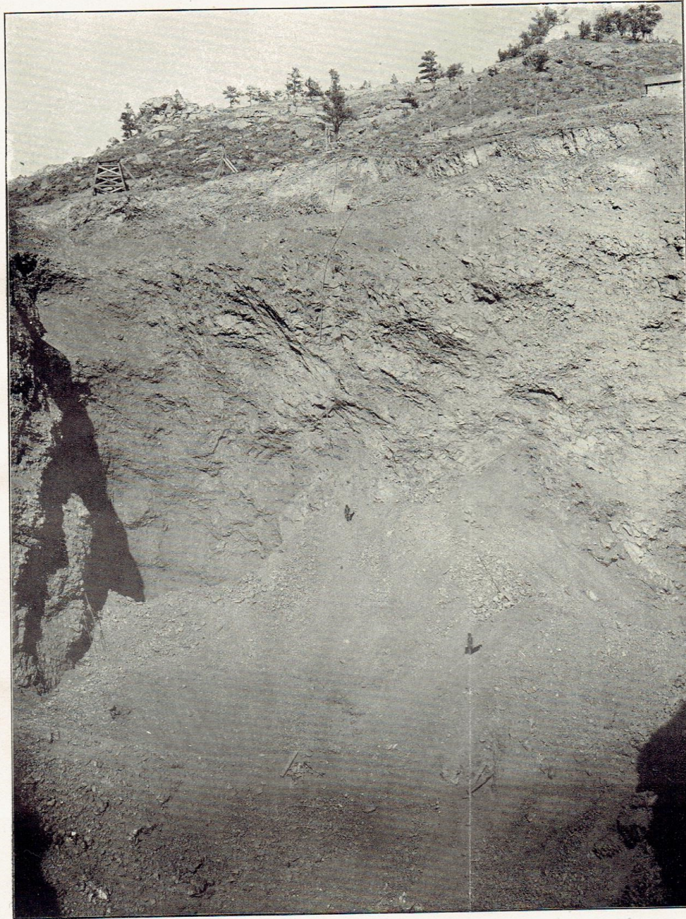
Interior of Pit No. 1, Showing One of the Mills.
