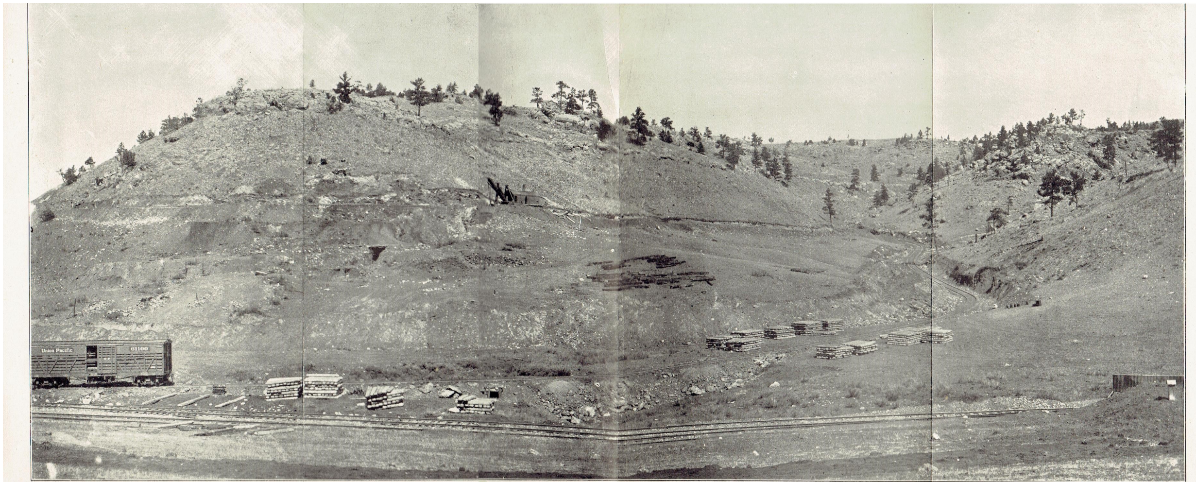
Showing First Operations at Sunrise. Stripping the First Open Pit Ore.
