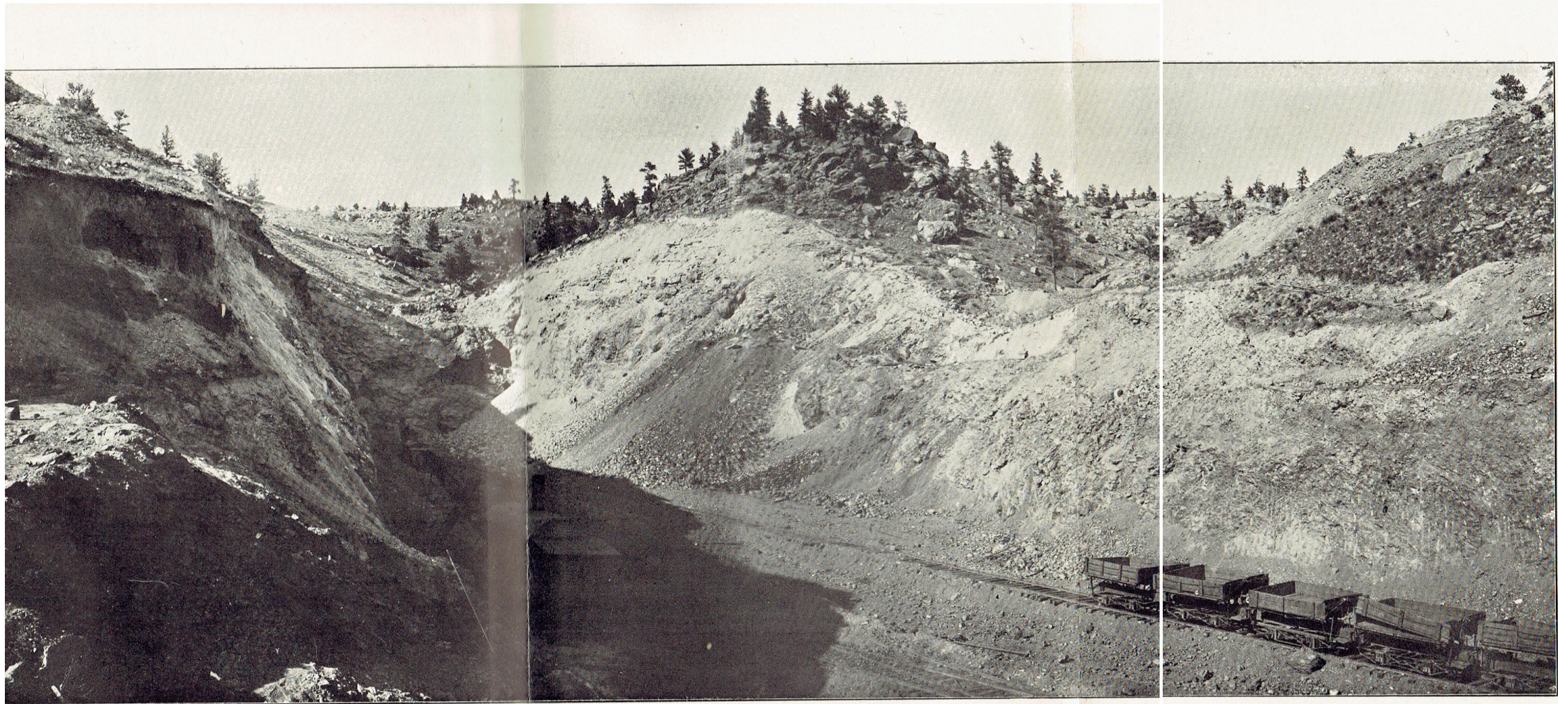
Operated with Steam Shovels. Extensive Shipping Operations Are Being Carried Forward on Both Sides of Pit.
